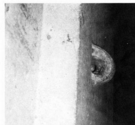
d. G 7140, Khafkhufu, tethering ring on south jamb to inner chapel, looking southwest
