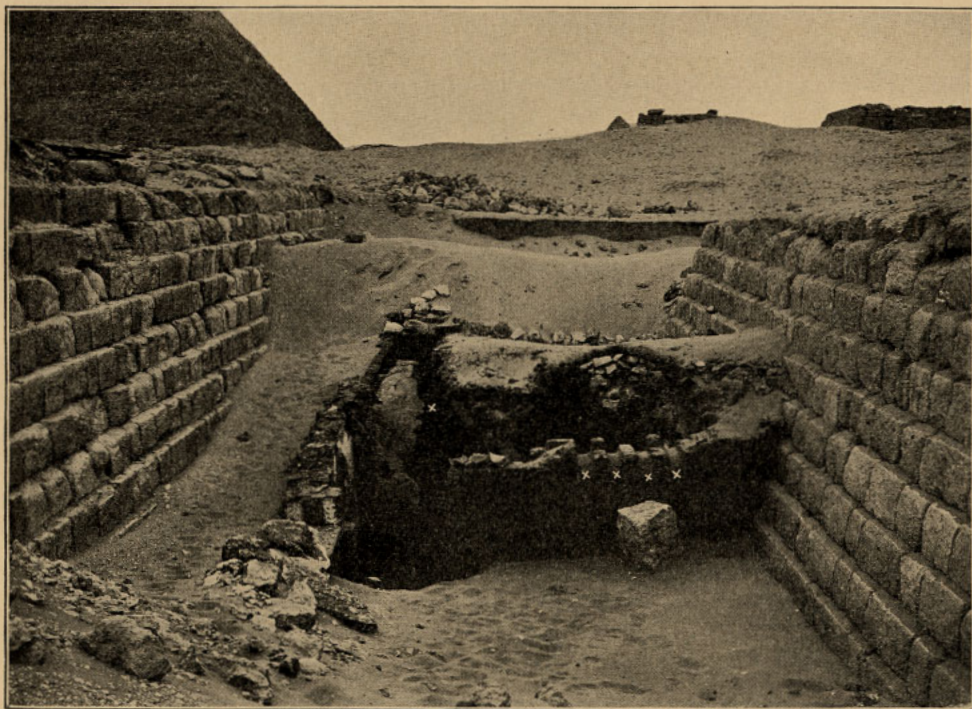
OFFERING CHAPEL, WITH BARREL-VAULT AND WINDOWS (X), OF A STONE MASTABA OF THE REIGN OF CHEOPS
